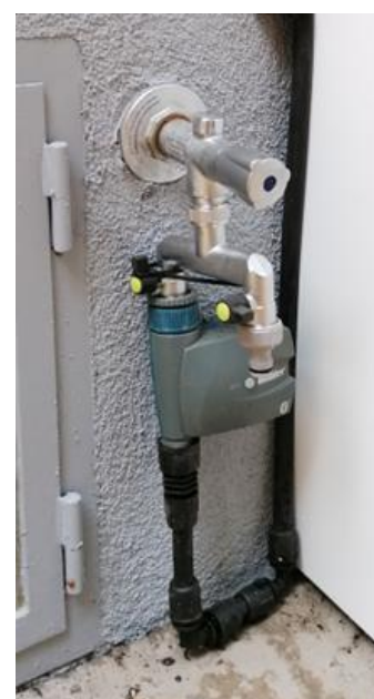
Figure 5: Control unit with solenoid valves in the interior (left) and with battery control unit outside (right) (Source: Dipl.-Ing. Ralf Dophiede e.U.)
